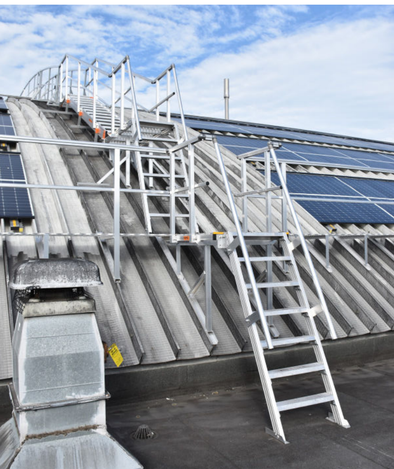
Two stage roof stair system designed to fit the slope of the dome roof line.
