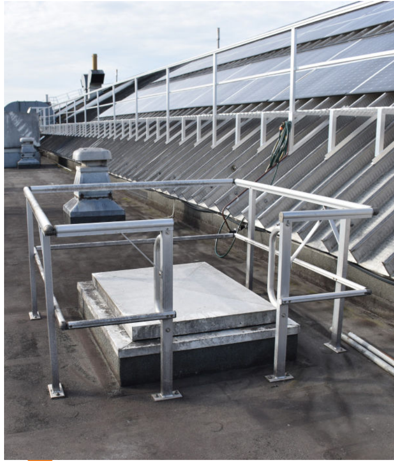
Guardrail and roof access hatch system.
