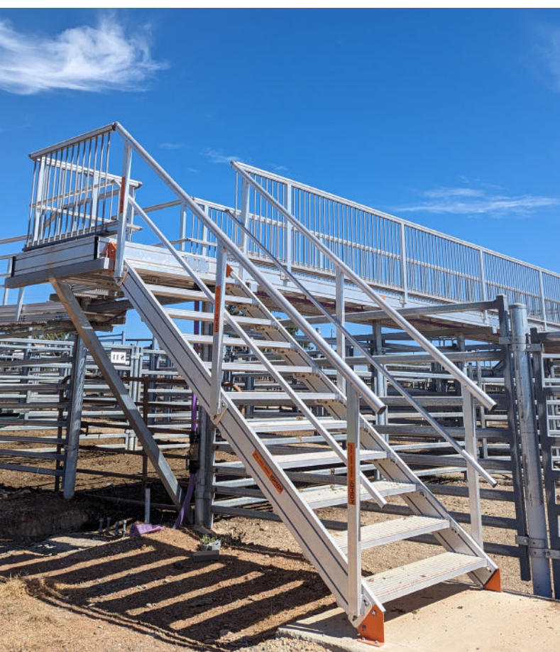
Public access stair system for safe access onto the walkway for viewing cattle.
