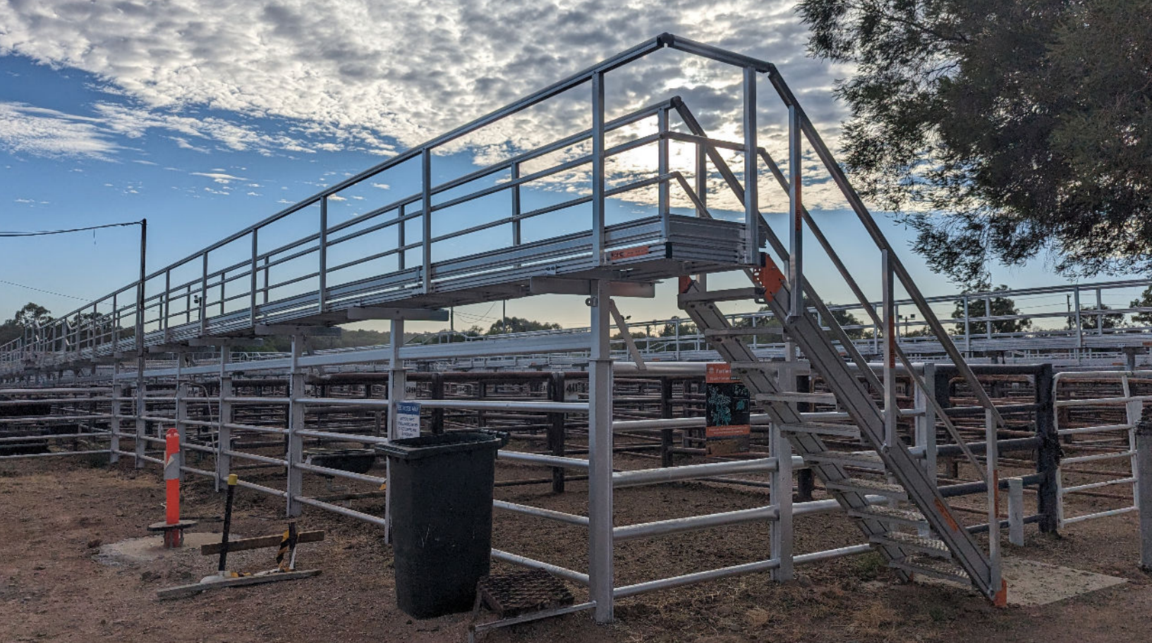
Auctioneers walkway & platform system retrofitted to existing yards with extended kick rail and guardrail each side.
