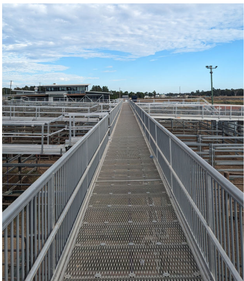
Public access walkway system with guardrail both sides.
