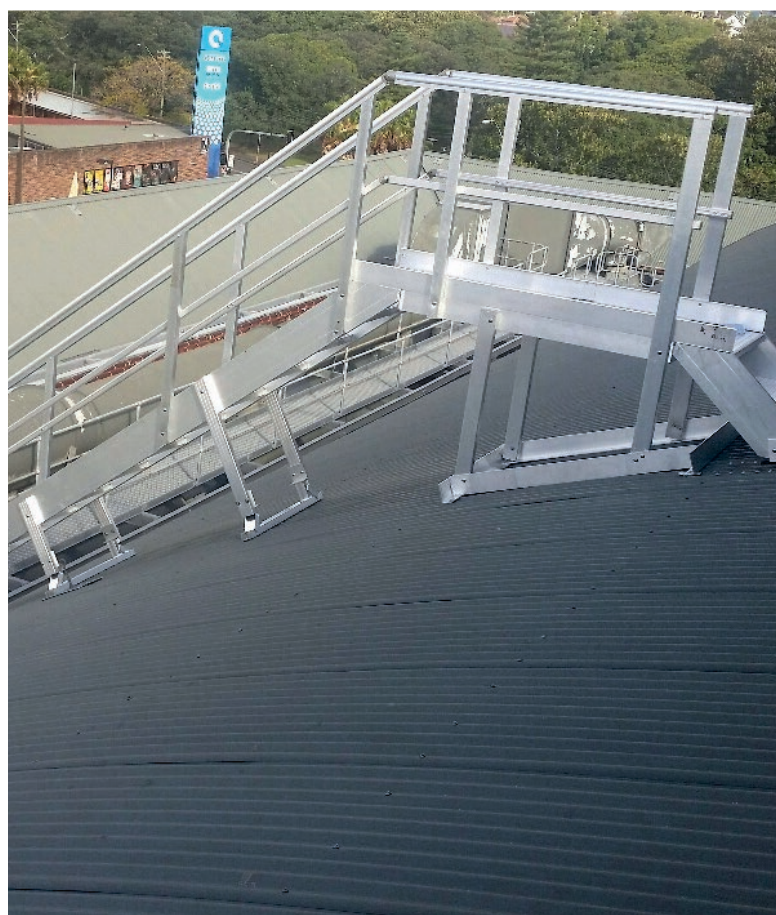
Stairway supported with adjustable supports made for ease of installation.
