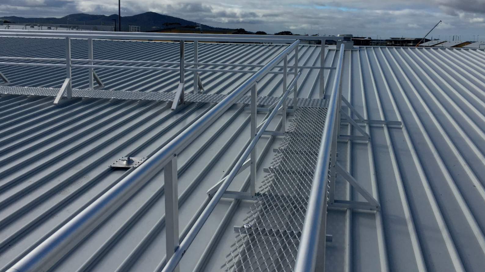
Walkway with double sided guardrail installed to ensure workers are safe and the roof is protected.
