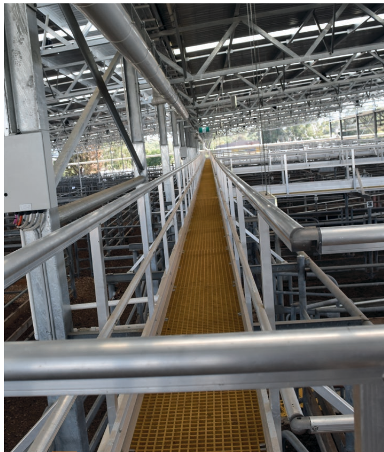
Quality workmanship by our qualified installation crew.
