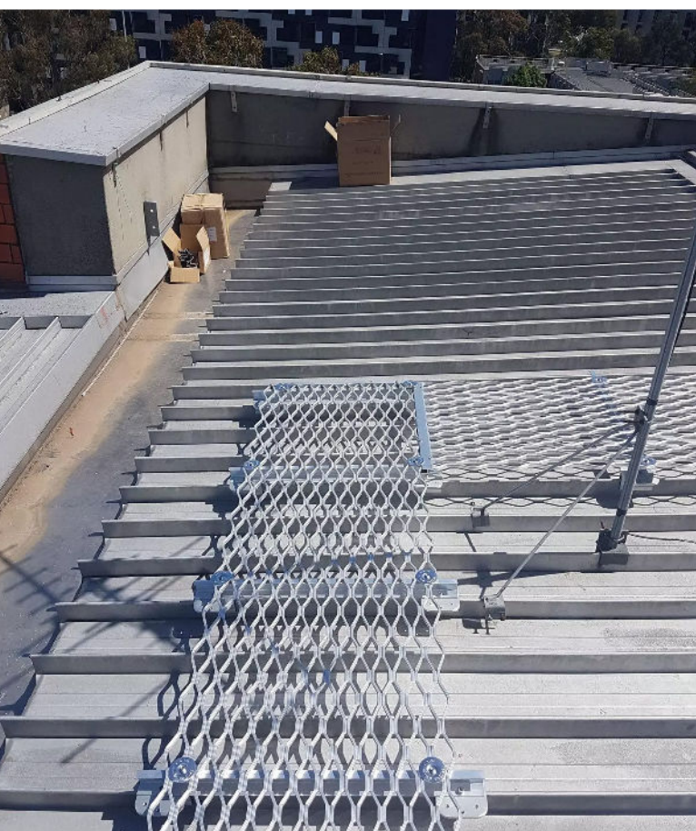
Anchor points in foreground for safe access to edge of roof.
