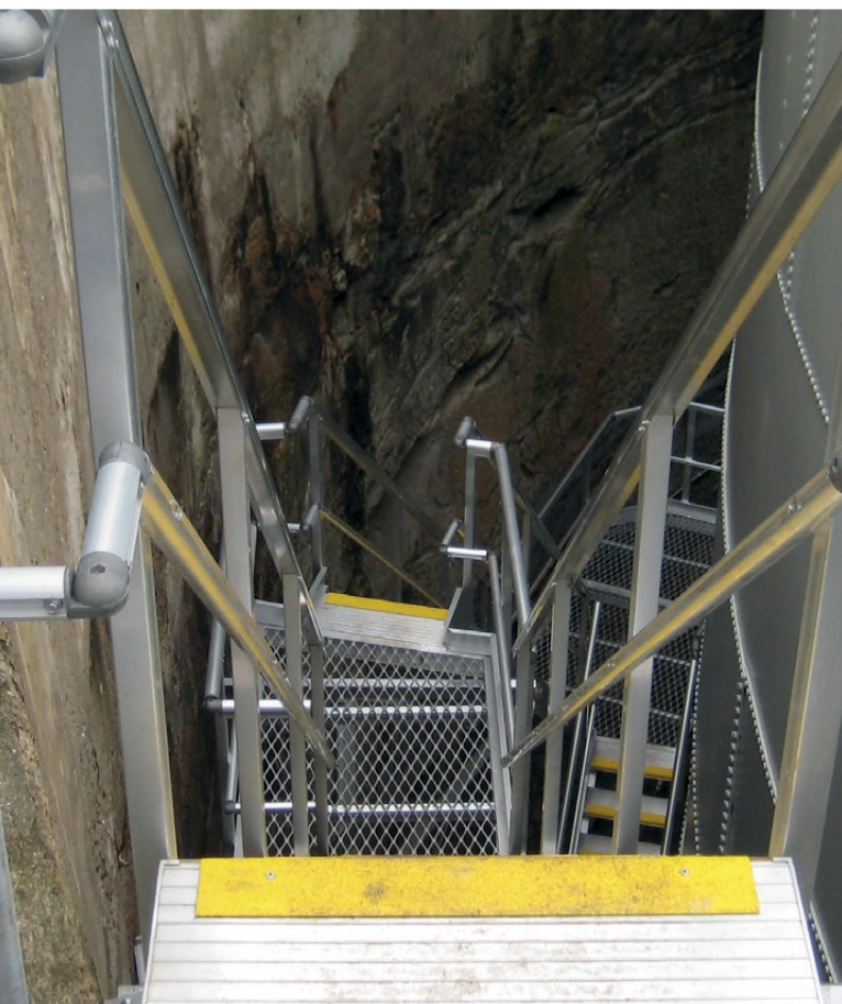
Display of quality skilled workmanship from one of our install team.
