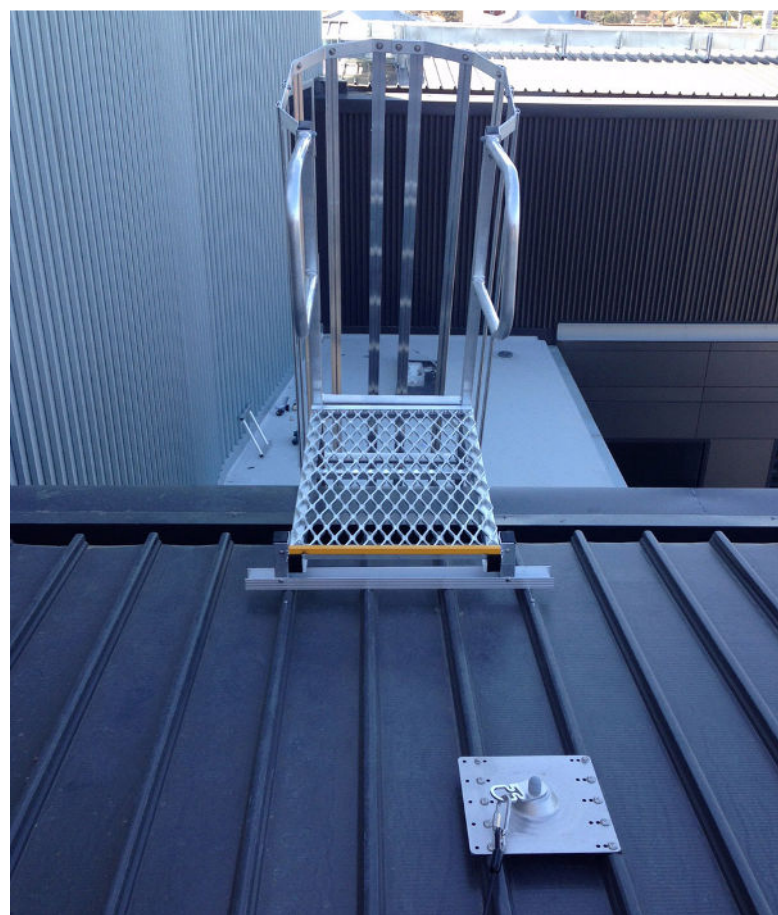
View from top of rung ladder system with anchor point for safe access onto the roof from ladder platform.
