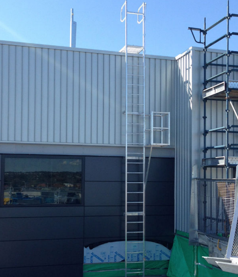
Rung ladder system with midway rest and vertical fall arrest line.
