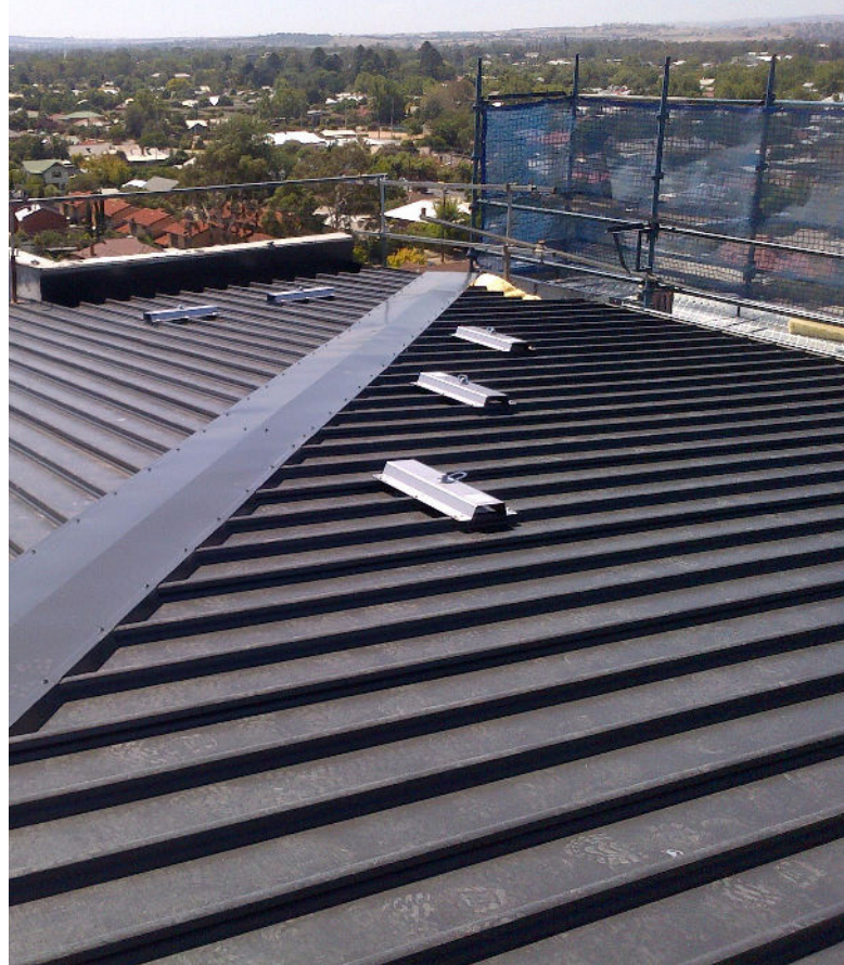
Anchor points installed for safe access to edge of roof.
