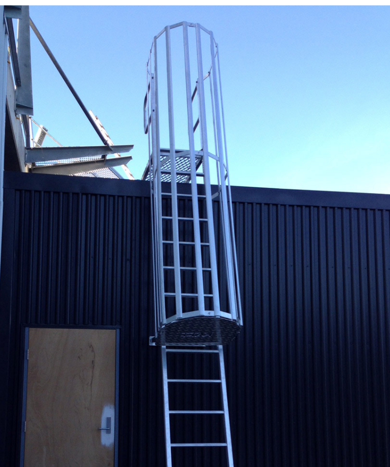
Rung ladder system with lockable ladder door preventing unauthorised access.
