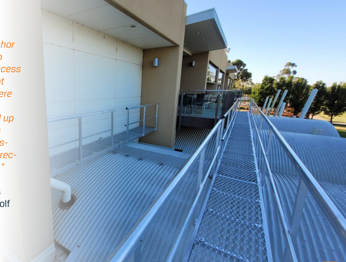
Extended walkway allowing access to the windows and other essential equipment.
