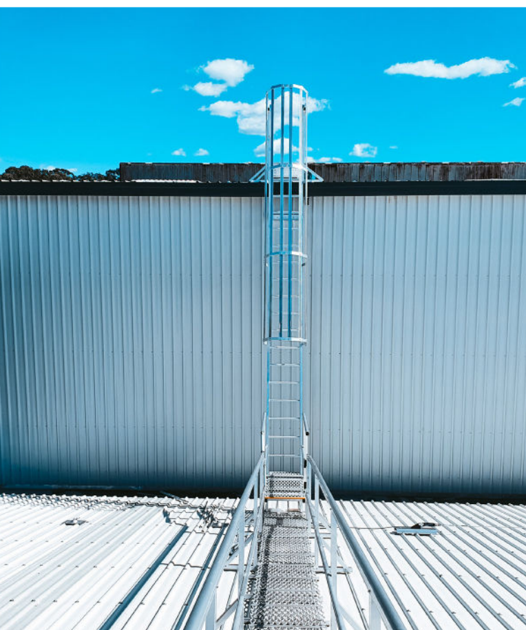
Access Cage ladder & landing platform
