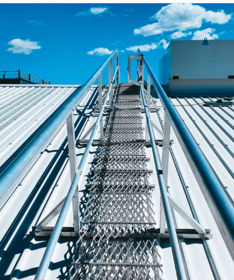
Walkway & Guardrail System with self-closing gate, another step to ensure safe at heights
