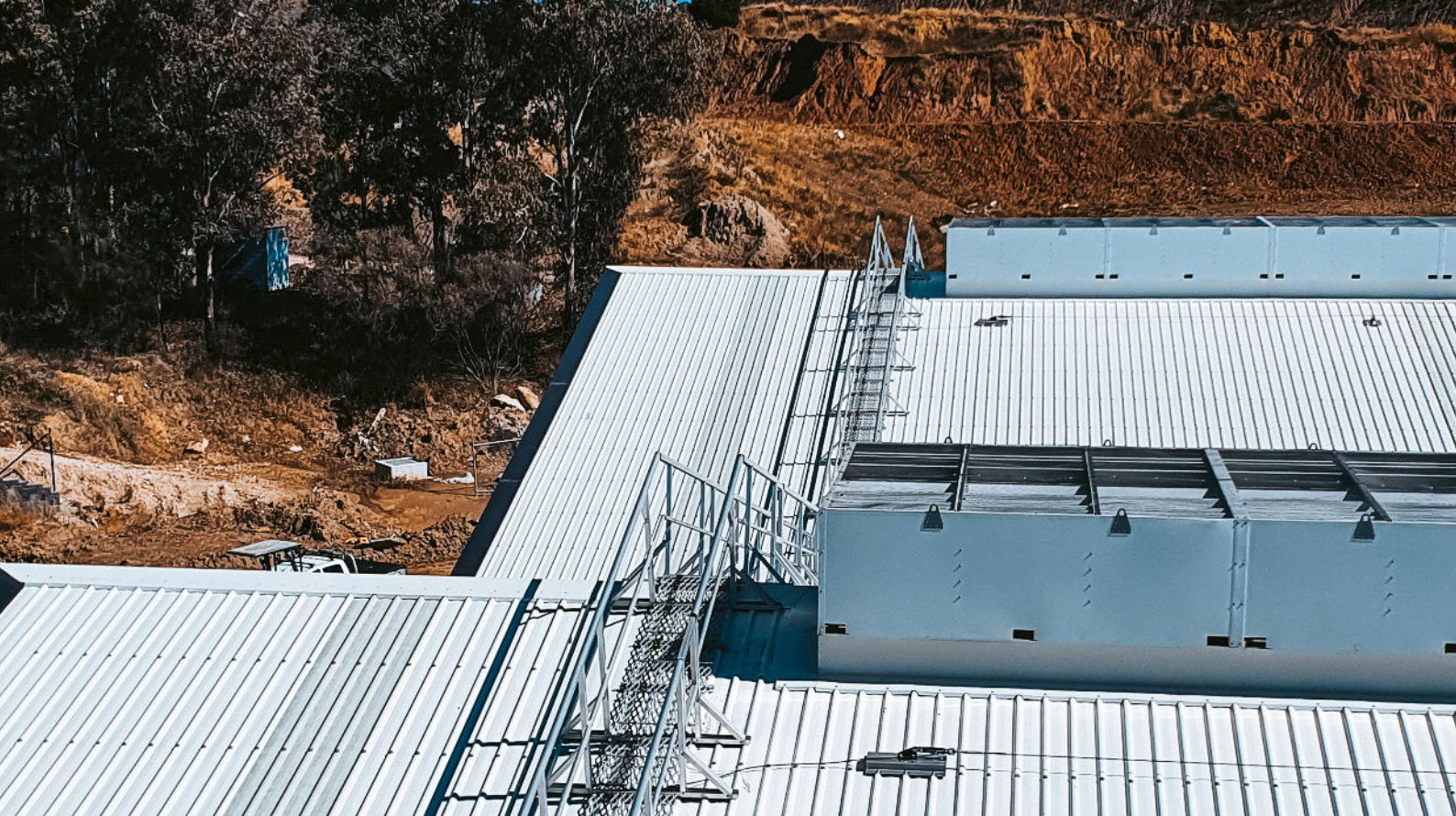
Walkway with double sided guardrail & self-closing gate installed to ensure workers are safe and the roof is protected.
