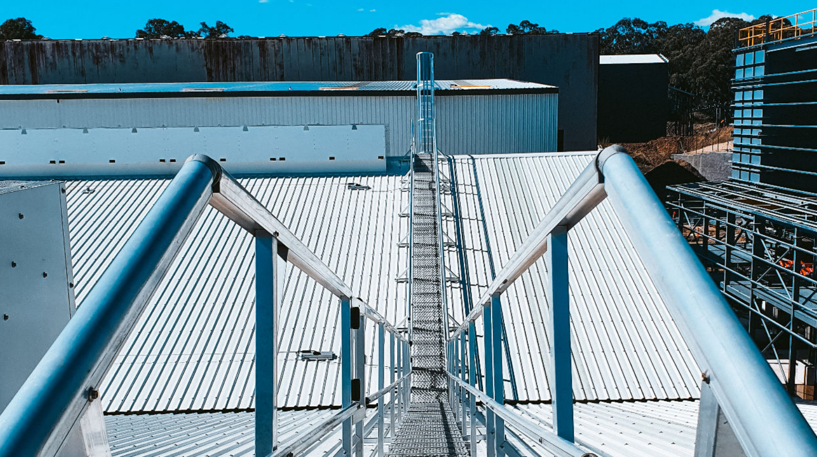
Walkway with double sided guardrail creating a designated safe path of access across the roof
