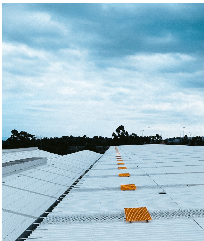
1.3km of static line & skylight protection to ensure the worker is in total restraint while accessing the box gutters
