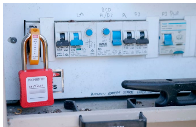
Image 11: Example of main electrical switch with lock
