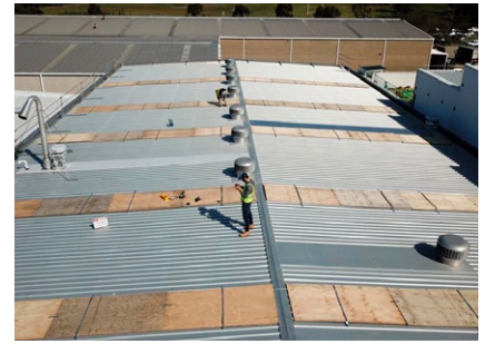
Images 8-10: Examples of physical barriers to manage risks of falling through skylights and brittle roof material.
