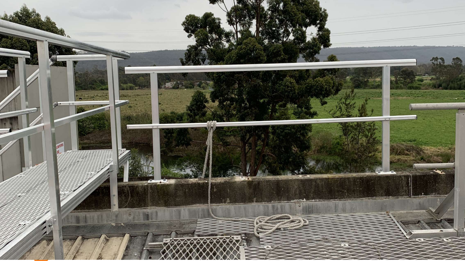
Guardrail & walkway system eliminating active fall edge
