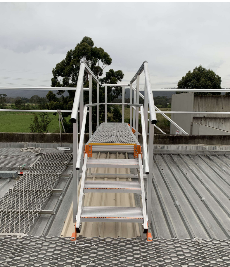
Stairway landing platform
