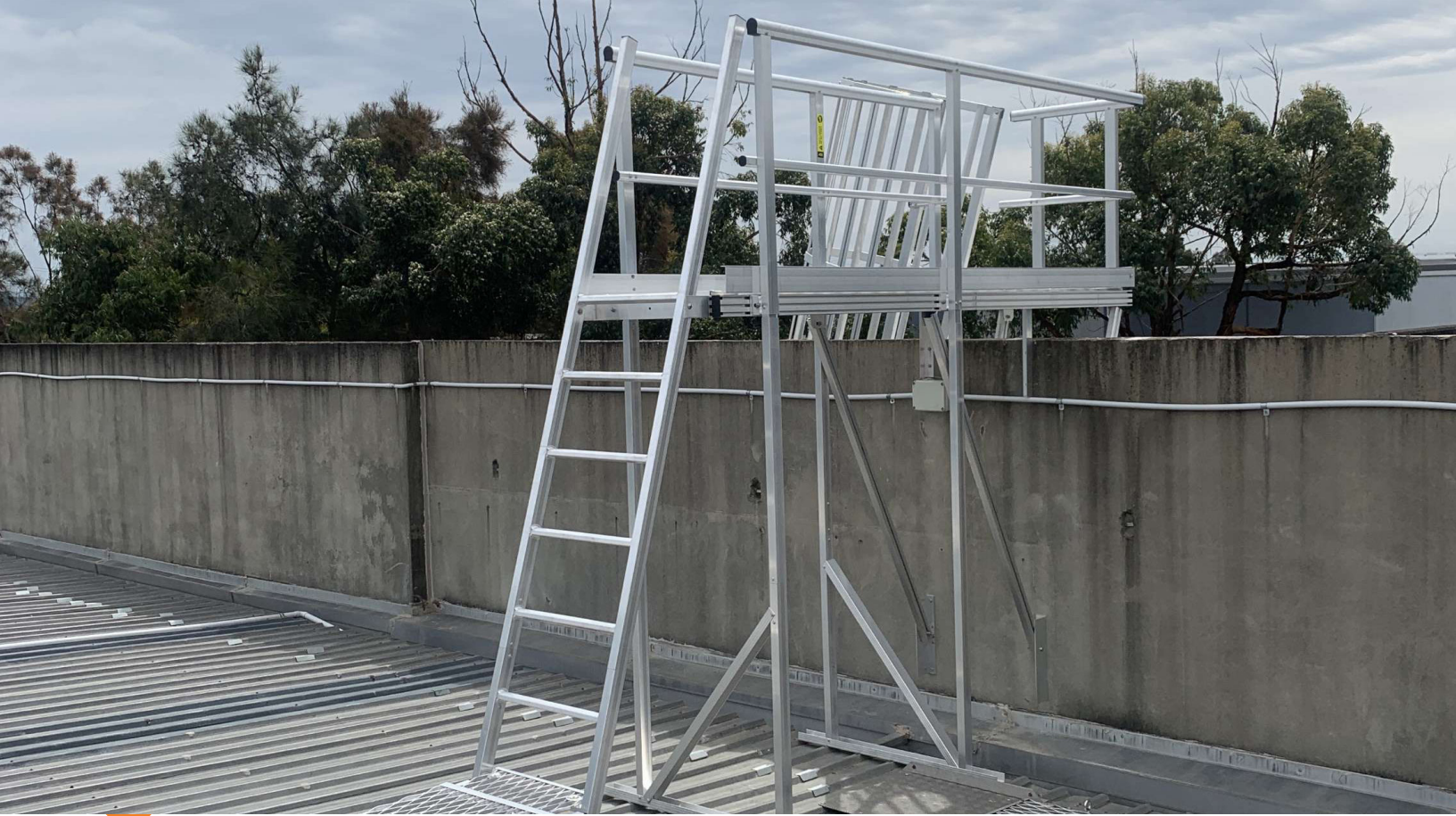
Landing platform and ladder system
