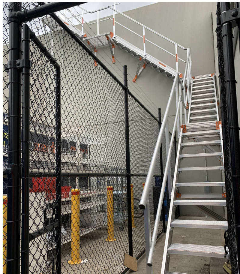
Security fence installed to ensure unauthorized access is eliminated.
