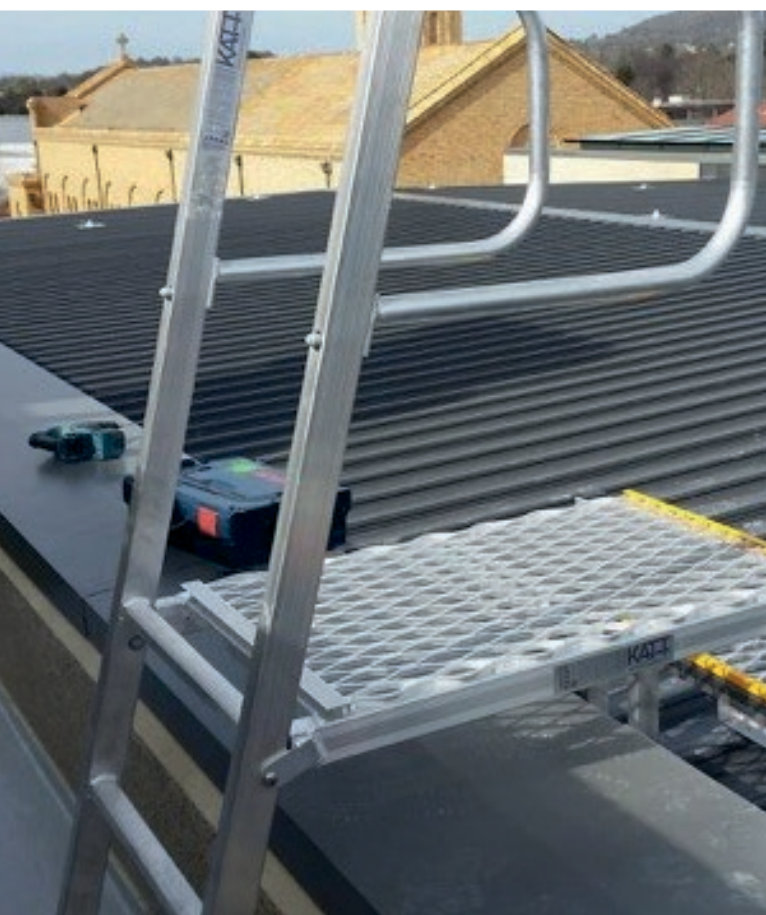
Photo displaying top landing platform.
